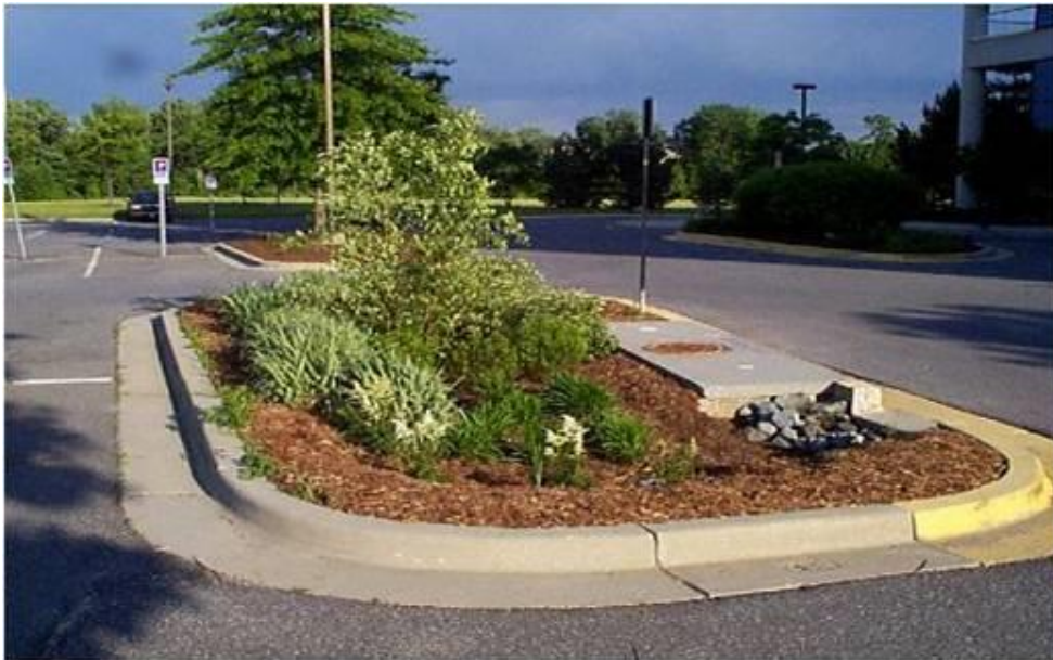
FIGURE 4-3 Bioretention in Parking Lot Island
